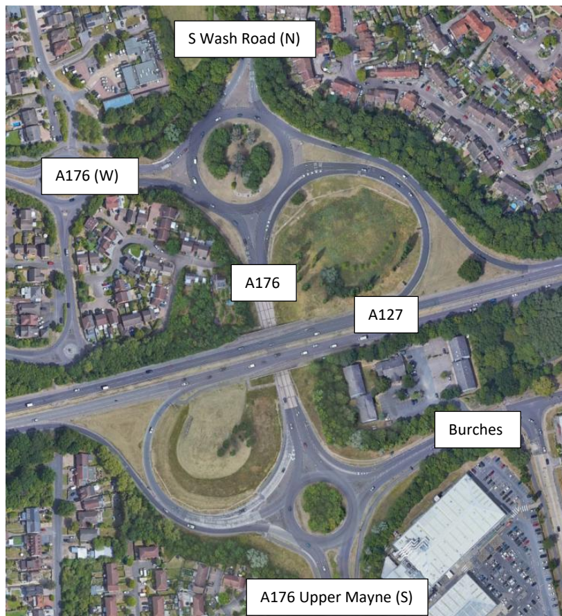
Image 7.20 A127 Southend Arterial Rd / A176 Noak Hill Rd roundabout
