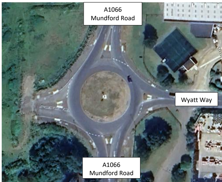
Image 7.33 A1066 Mundford Road / Wyatt Way roundabout
