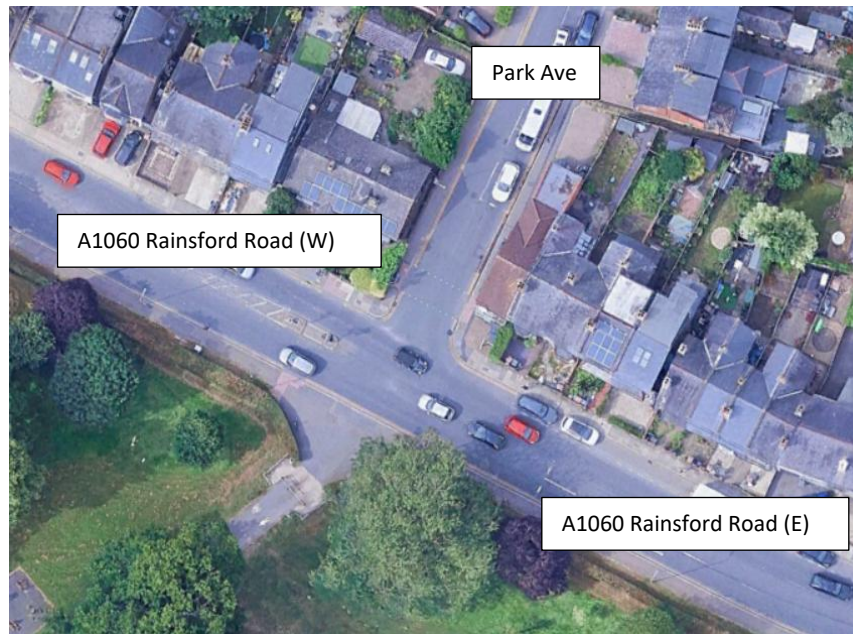
Image 7.60 A1060 Rainsford Rd / Park Avenue
