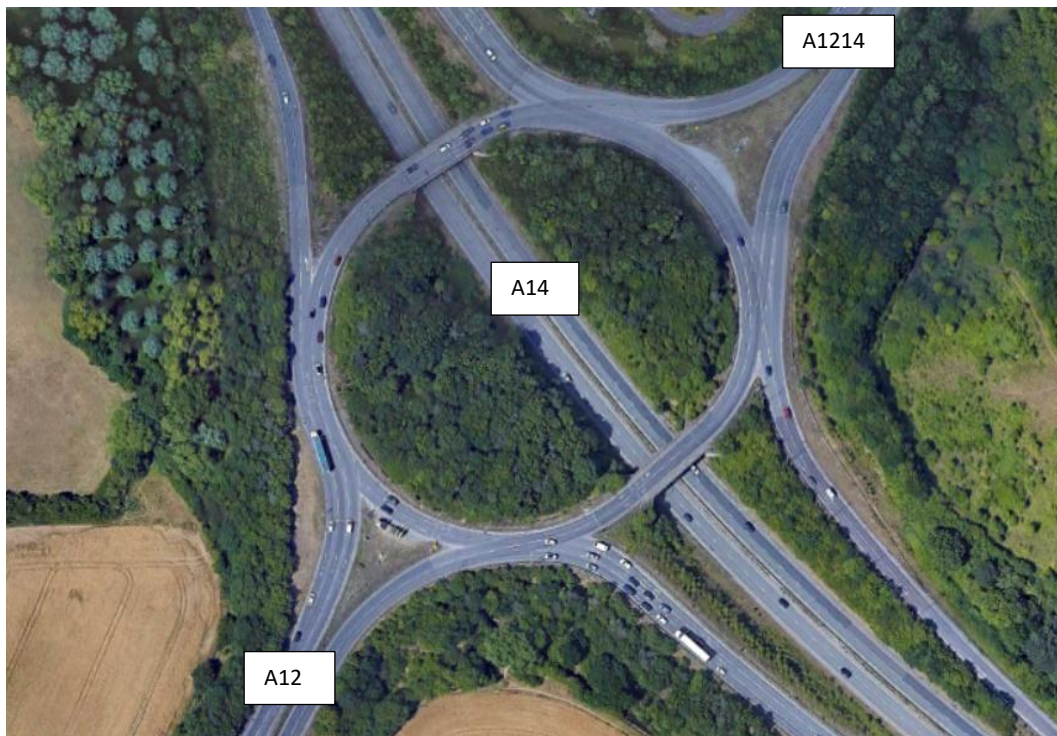
Image 7.6 A14 J55 Copdock Interchange
